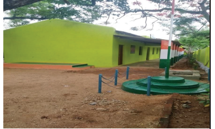
School Building Painting completed at Govt. Higher Primary School Chitraiahnahatty, Challakere Taluk, Chitradurga Dist.
